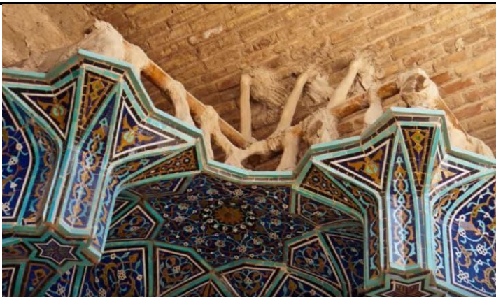
Fig. 5.1. Sazu, the traditional rope used for hanging layers of muqarnas (Source: Shakouiri Saeid)
