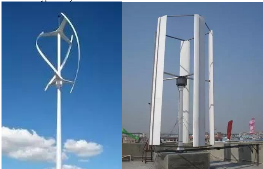
Figure 1. Vertical axle wind generator.
