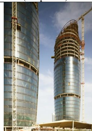
Fig 27 Almost finished installing the curtain wall (Yacoubian 2020)
