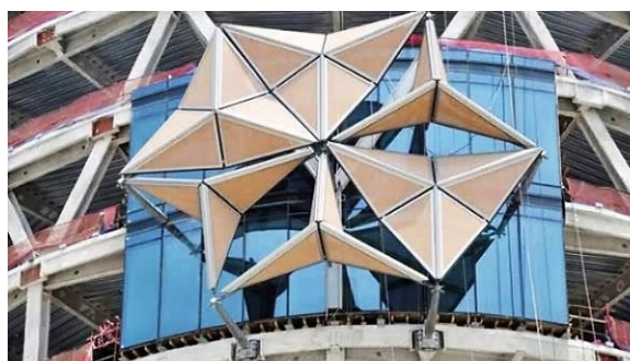
Fig 33 The mashrabiya mechanism test on site (MGS 2020)
