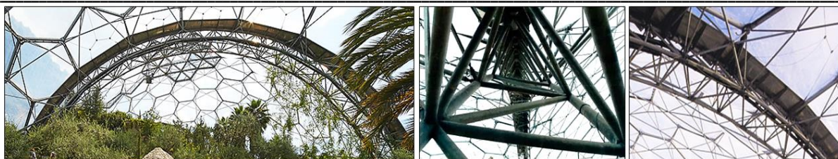
Fig 45 Steel arches between geodesic domes (Knebel and others 2001) (Eden-Project-Co 2020)
