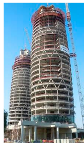
Fig 25 Tower construction work (Arup 2014)
