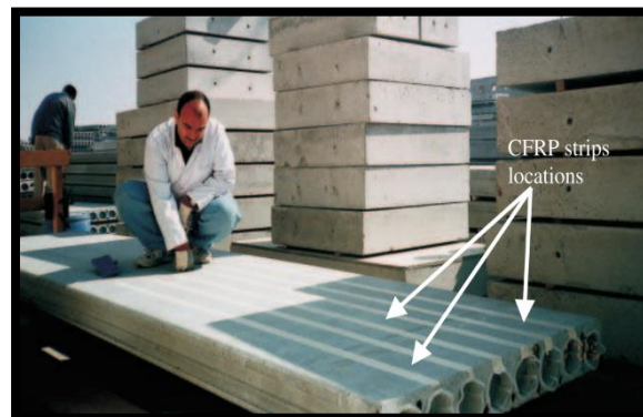
Fig.1 Marked locations of the CFRP strips on Slab
