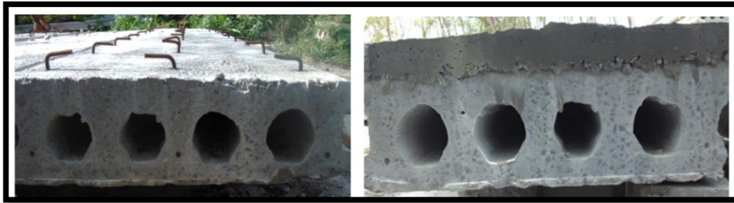
Fig.5 Hollow Core Slabs with Bonded Overlay
