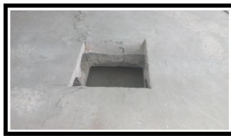
Fig.6 hollow core slab content holes
