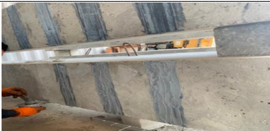
Figure 3: EBR strengthening.
