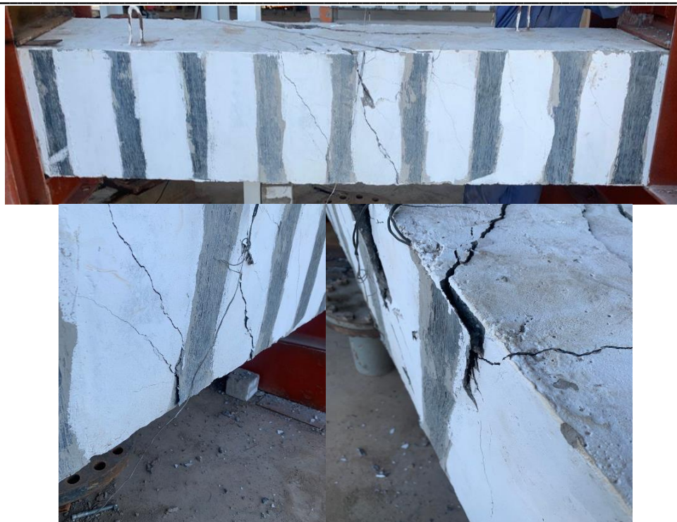
Figure 7: Strengthened beam ES-1 failure and crack configuration
