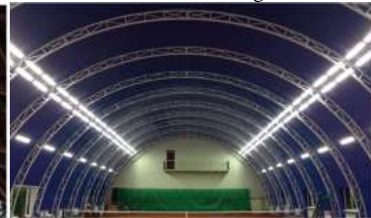
Fig.4 Arched coating of the gym.
