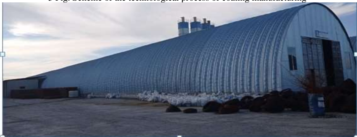
Fig. 6. Arched coating made of profiled sheet.
