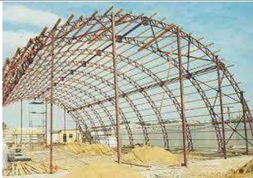
Fig.1 Installation of through arches
