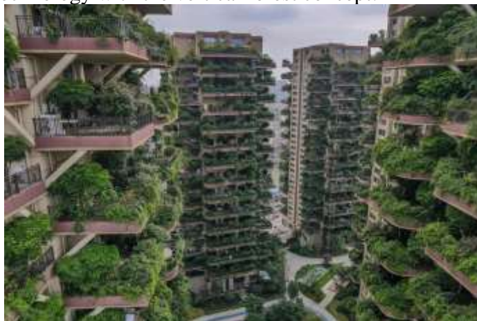
Figure (3): Vertical Forest Housing Project in China
