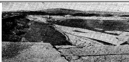
Fig. 4. View of the lower San Fernando dam after the earthquake [7].
