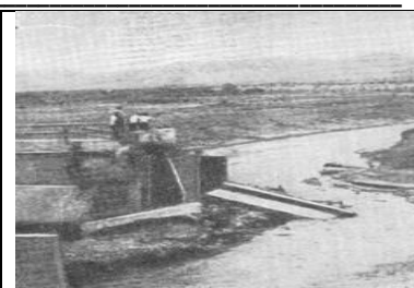
Fig.5. Collapsed earthen dam at Rogers Dam [10]
