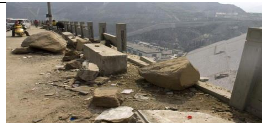
Fig. 9. Fragments of damage to the Zipingpu dam during an earthquake in Sichuan[8]
